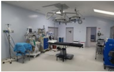
Renovation of Operating Theatre
